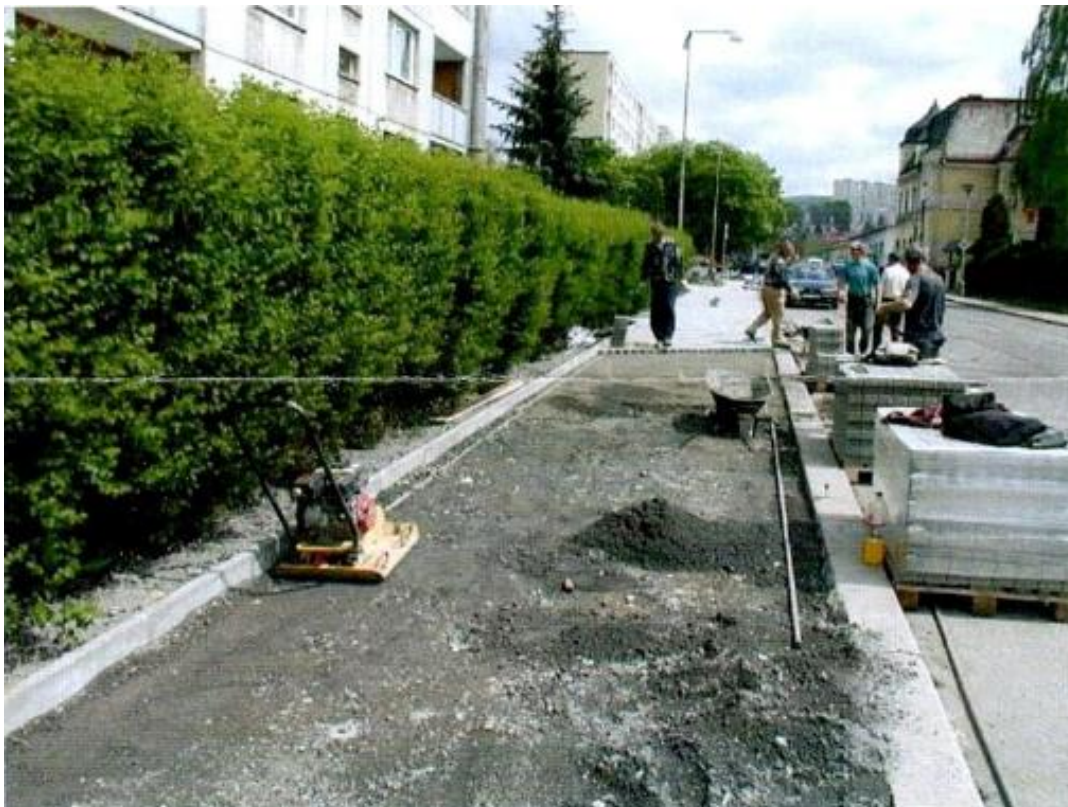
Photo 3: Promotion of use of mixed fly ash and bottom ash as undercover for sidewalks in the Czech Republic. Levels of PCDD/Fs in this mixture are about 0.05 – 0.1 ppb in WHO-TEQ. (Source: Letter sent by company Termizo, operating MWI in Liberec to mayors in the region)
